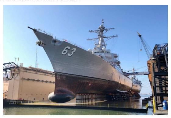
Double docking of USS Decatur (DDG 73) and USS Stethem (DDG 63) in BAE Systems - Ship Repair's dry dock.
